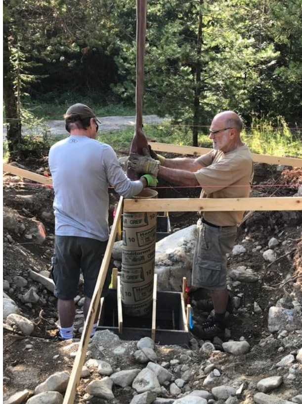
Warren and Ernie helping with the cement pour.
