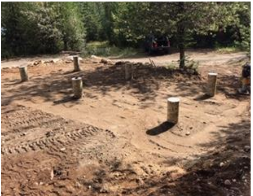
Compacted and ready for construction.
