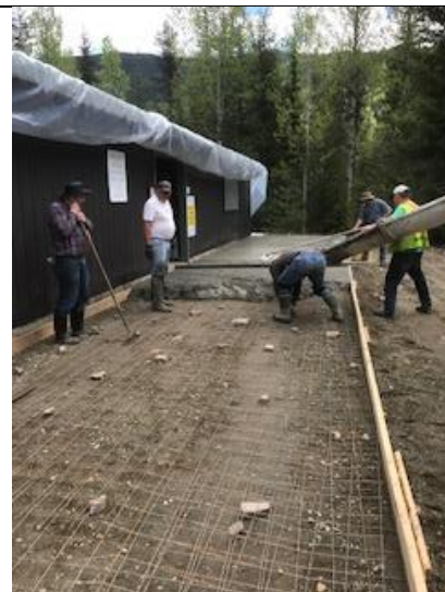
Prepping the pad.
