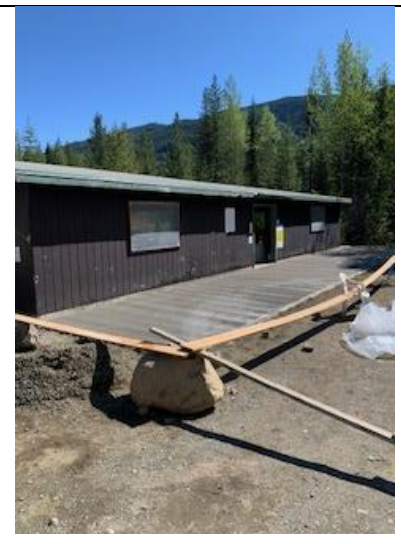
Concrete poured on new pad.
