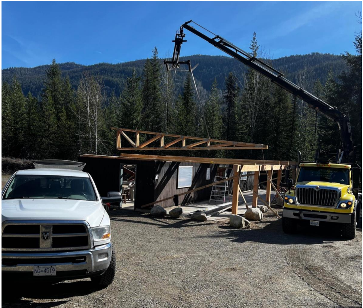
Home Hardware Donated the Liftruck for the Beams and Trusses:
