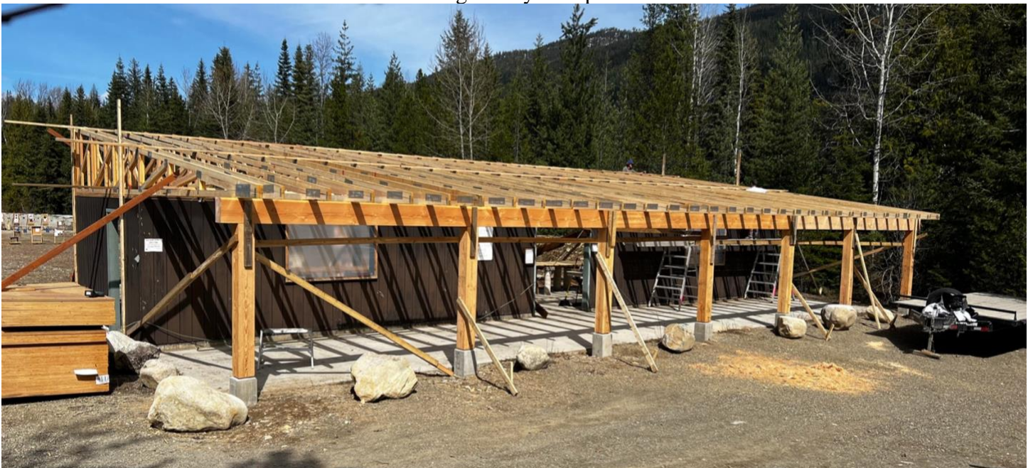
Framing Nearly Complete:
